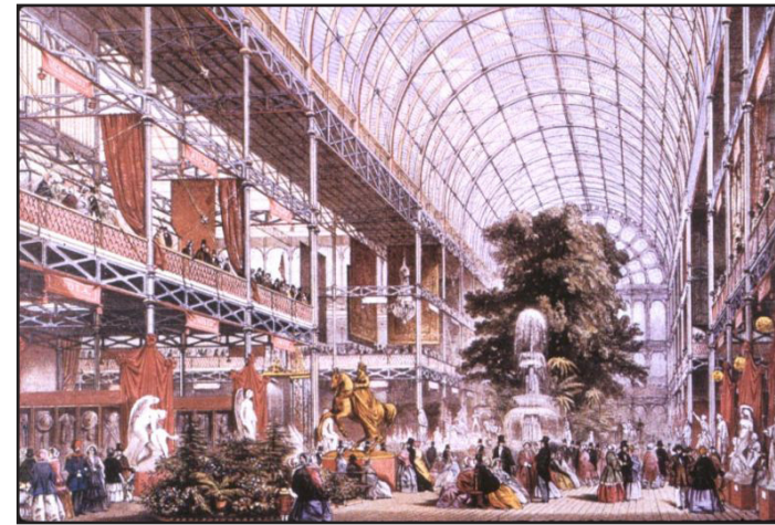
148. Joseph Paxton, Crystal Palace , London, 1850-51. Cast iron, wrought iron, and glass. Engraving. Drawings Collection, Royal Institute of British Architects. London. The Crystal Palace was 1850 feet (564 m) long (perhaps an architect’s pun on the year in which it was built) and 400 feet (122 m) wide. It covered an area of 18 acres (7.3 ha, enclosed 33 million cubic feet (934,000 m 3 ) of space (the largest enclosed space up to that time), and contained more than 10,000 exhibits of technology and handicrafts from all over the world. In 1936 the it was destroyed in a fire.
