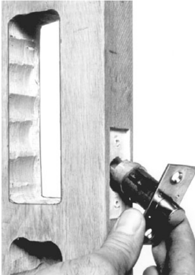
Figure 18.49 Preso-Matic installation, Step 3.
