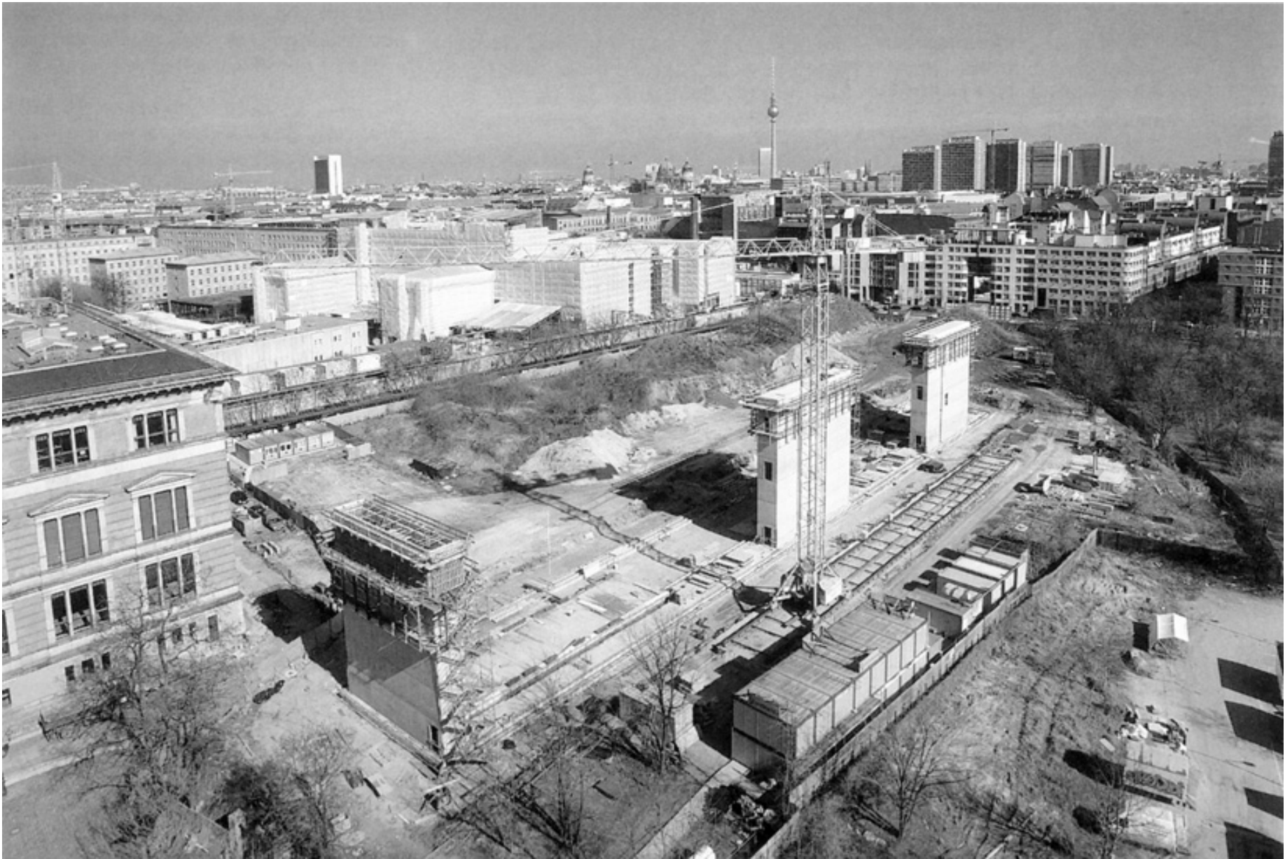
Construction site 1999, with winning entry by Zumthor from the Competition in 1993
