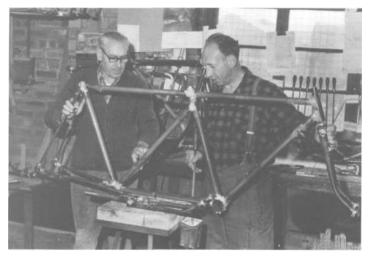
Figure 8-1: Jack (left) and Norman Taylor inspect a newly brazed tandem frame.
