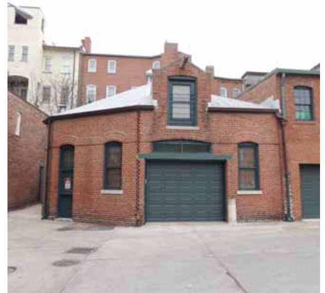
This angled stable building in Hillyer Court in the Dupont Circle Historic District, built in 1903, was designed to align with the irregular alleyway.
