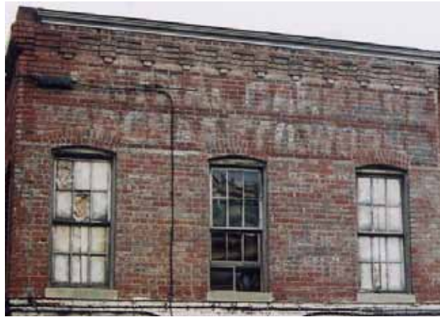
Detail of Beuchert's Blacksmith Shop, 443 (Rear) I Street, NW (1912), showing ghosting of business advertisement at cornice line.
