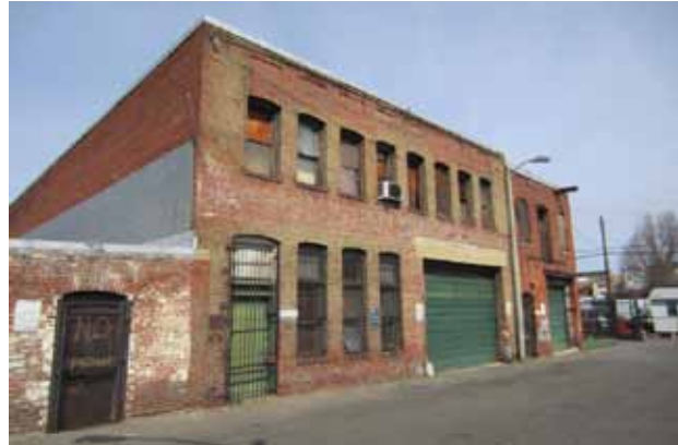
Warrington Motor Car Company, 1349 Cedar Court, NW (1919), U Street Historic District
