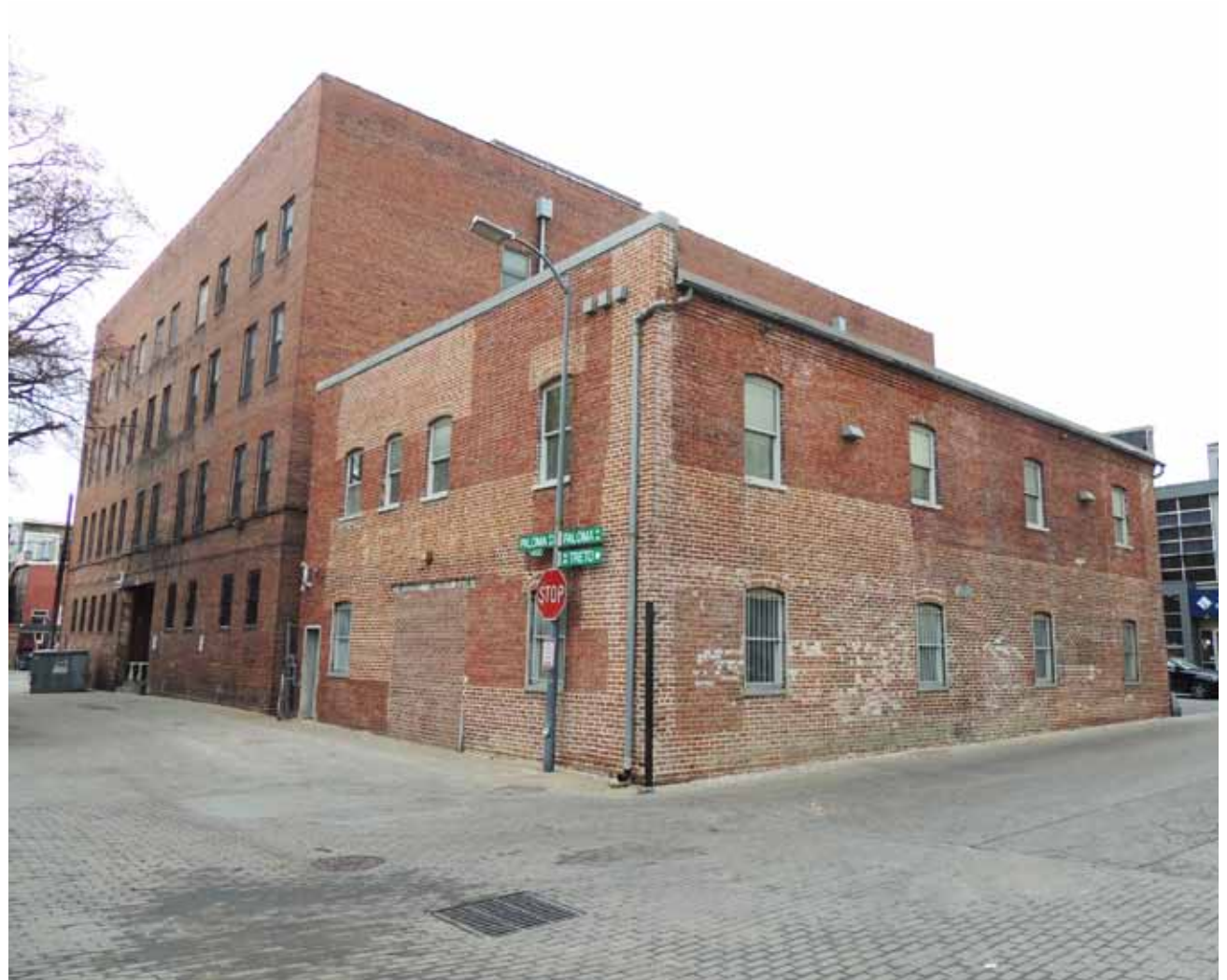
Dr. Coblentz Garage, 1432 (Rear) U Street, NW
