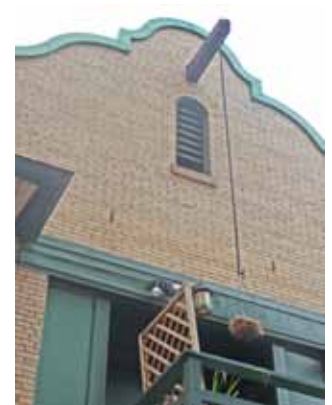
Block and tackle at Walsh Stable, 1523 (Rear) 22nd Street, NW
