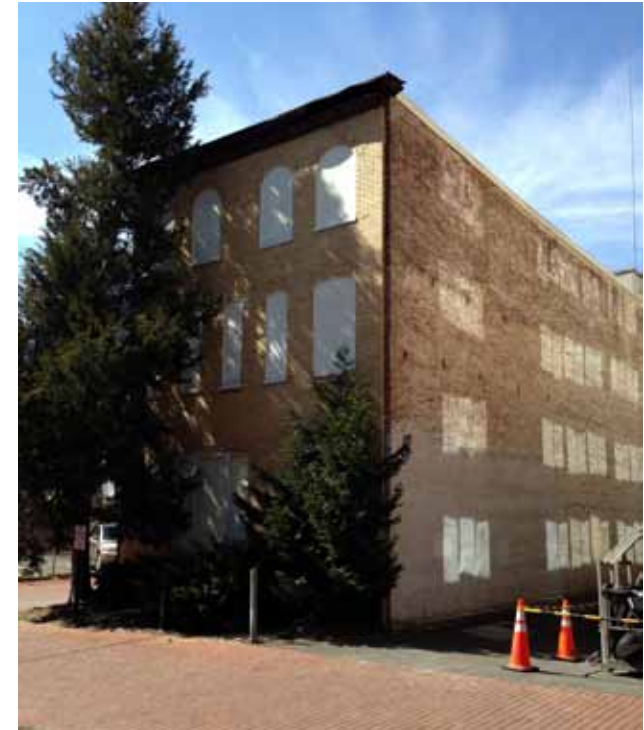
Snow's Court Stable, Foggy Bottom Historic District
