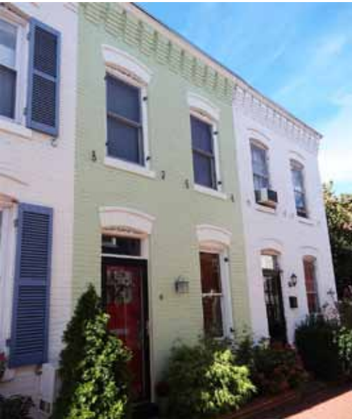
Alley dwellings in Terrace Court, NE (1889), Capitol Hill Historic District
