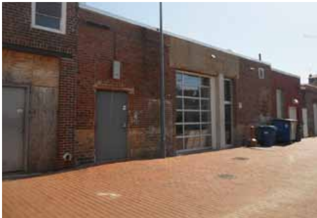
Printing Shop, 1232 (Rear) 9th Street, NW (1946), Blagden Alley/Naylor Court Historic District
