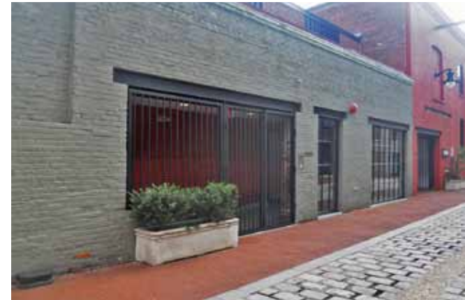
Mid-20th-century warehouse, 3340 Cady's Alley, NW Georgetown Historic District
