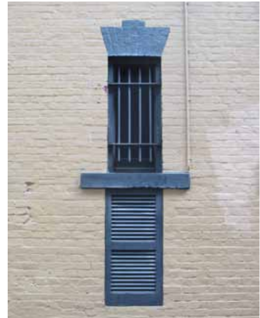
Detail of stall window on stable in Green Court
