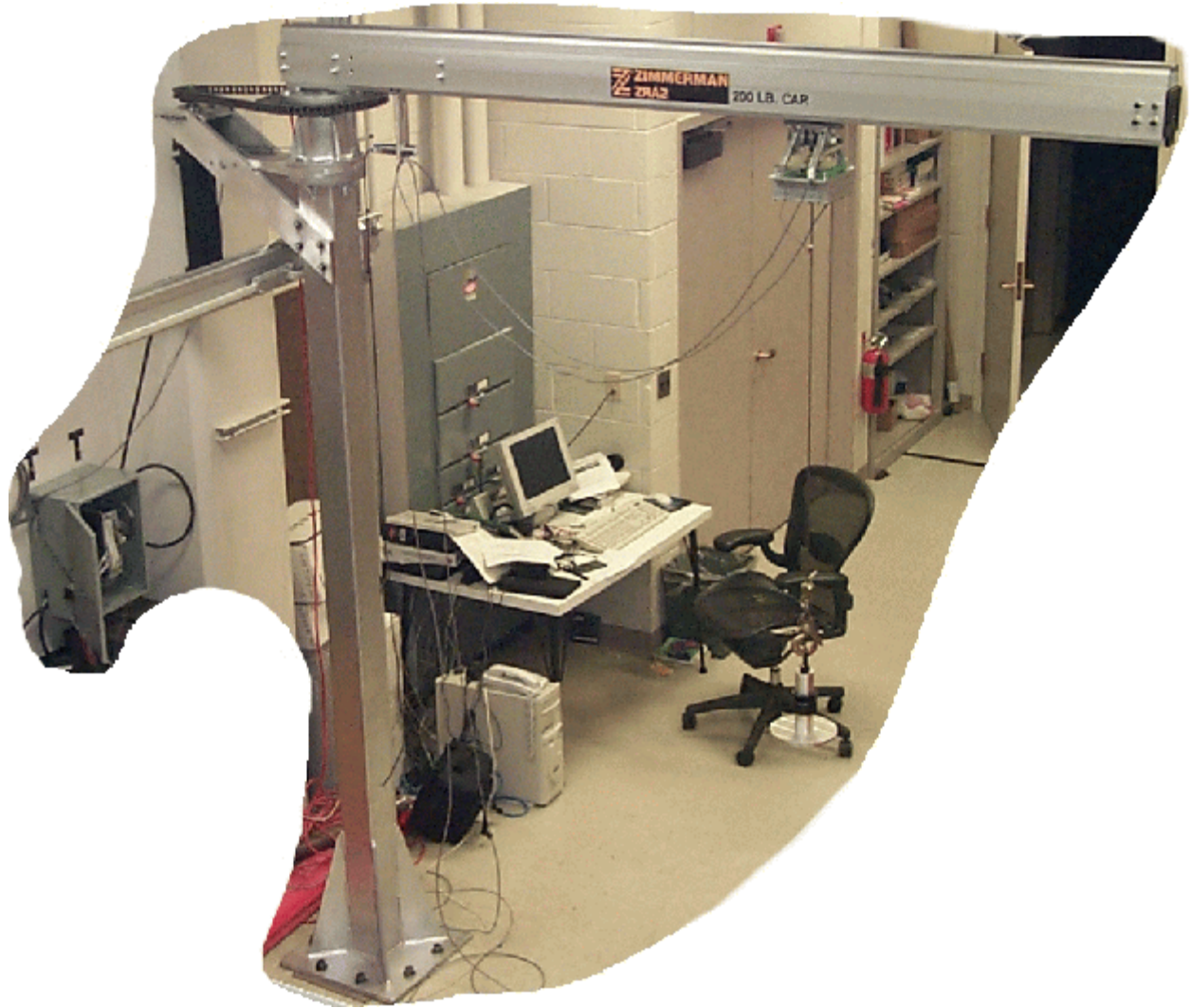
Figure 2.26 Completed Platform for an Intelligent Power Assist Jib Crane
