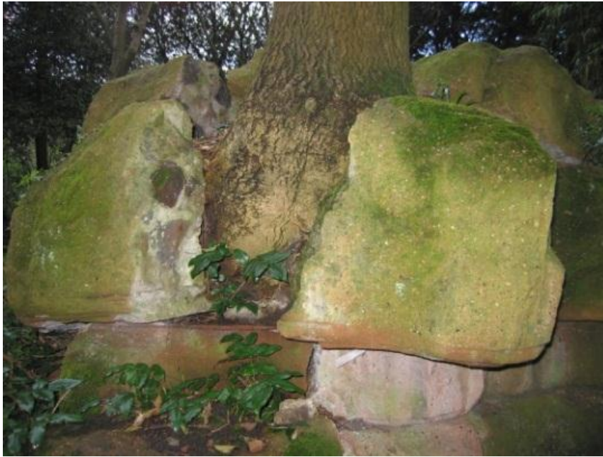
Figure 17 Tree roots damage the Pulhamite in places.
