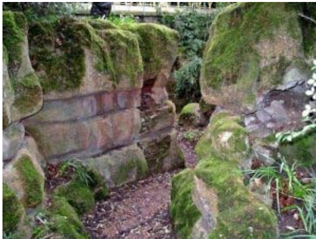
Fig 6 - An area of cement has broken away to reveal its brick base
