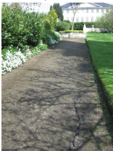
Figure 21 An appropriate replacement will be needed for cracked tarmac.
