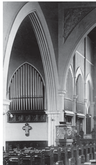
Original 1902 Kimball façade
