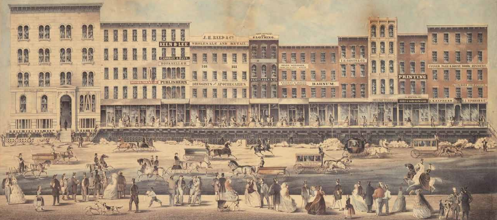
Workers raise the Briggs House in Chicago.
