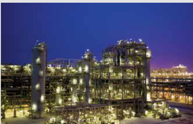
Pearl GTL, Qatar 140,000 bpd of GTL Products
