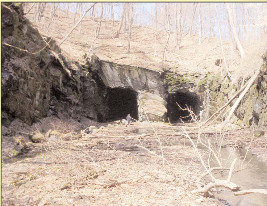
Manunka Chunk Tunnels South face today.
