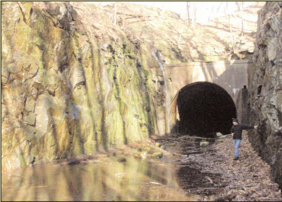
South face of Oxford Tunnel Photo from author's collection
