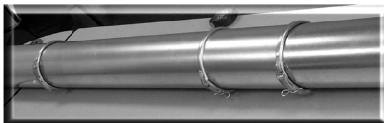
Cut piece of pipe put O-ring on cut pipe, slide nipple over
