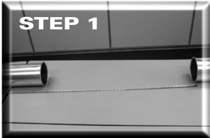
Measure distance to be spanned.
