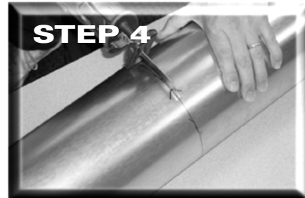
Drill access hole then cut with saw
