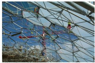
1.08 Installation of the ETFE pillows. Source: <http://www.eden-happenings.com/biome-con.htm>
