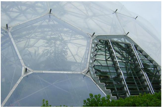
1.11 Up-close look at the transparent glazing of the ETFE pillows and ventilation. Each hexagon (or pentagon) is a slightly different size, allowing the structure to better conform to the site. Source: <a href="http://www.rpcurnow.force9.co.uk/photos/hols\_2004/dscn2214\_800.jpg">http://www.rpcurnow.force9.co.uk/photos/hols\_2004/dscn2214\_800.jpg</a>
