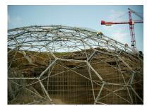
1.12 Construction of the steel hexagonal bracing Source: <http://www.eden-happenings. com/biome-con.htm>
