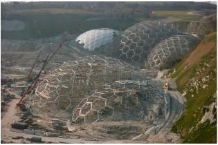
1.07 The domes under construction against one of the side walls of the old clay quarry. Source: <a href="http://www.eden-happenings.com/biome-con.htm">http://www.eden-happenings.com/biome-con.htm</a>
