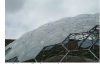
1.13 Specially designed connectors were designed to connect the ETFE pillow membranes to the steel structure. Source: <a href="http://www.eden-happenings.com/biome-con.htm">http://www.eden-happenings.com/biome-con.htm</a>
