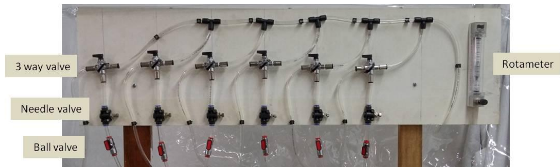
Figure 11. The valves system.
