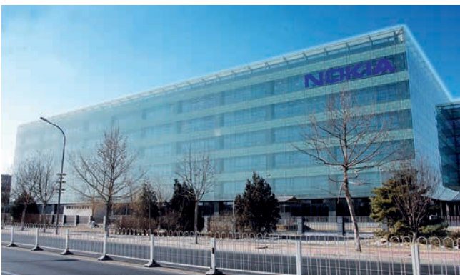
Nokia Headquarters Business Building, Beijing, China
