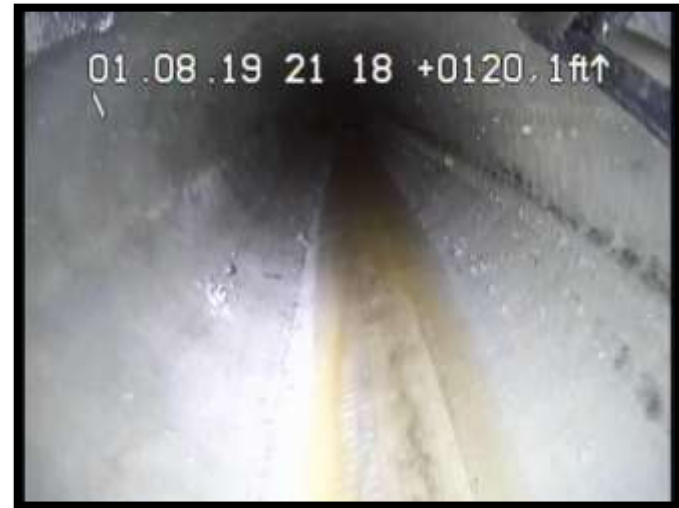
Lift in CIPP Robotically Cut Out
