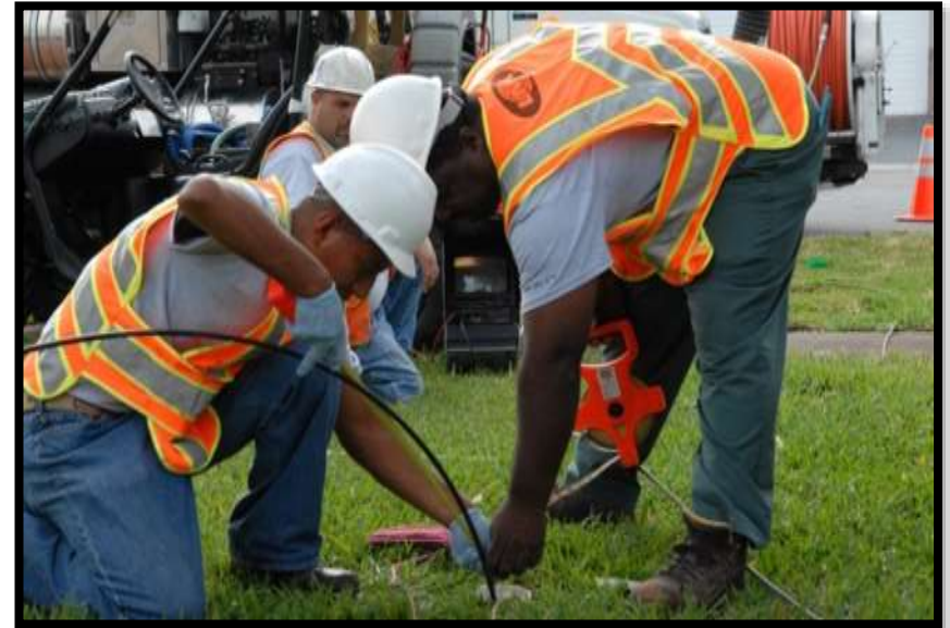
Measuring Lateral Pipe for Exact Liner Length
