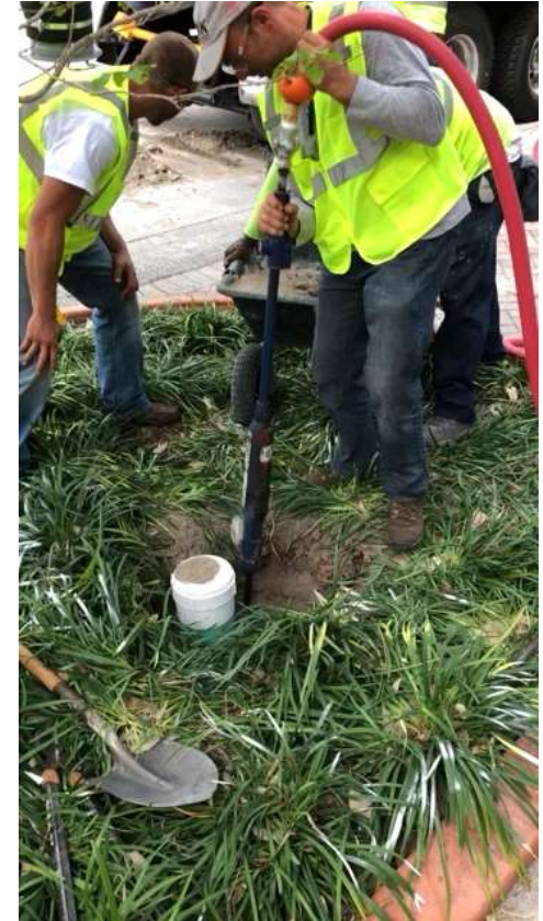
Compacting Trench Fill
