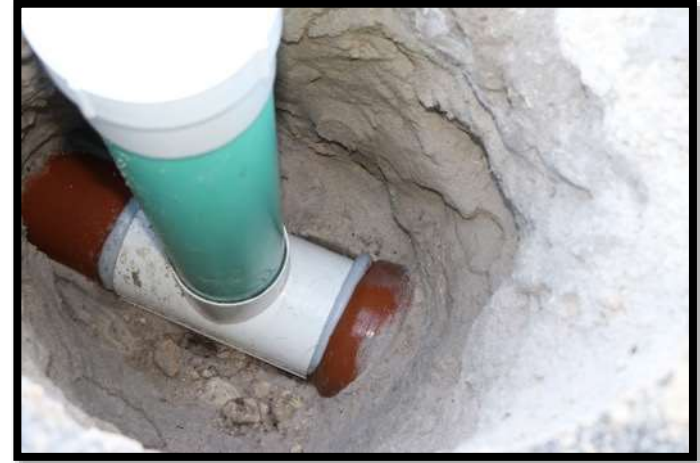
Vacuum Excavated Cleanout
