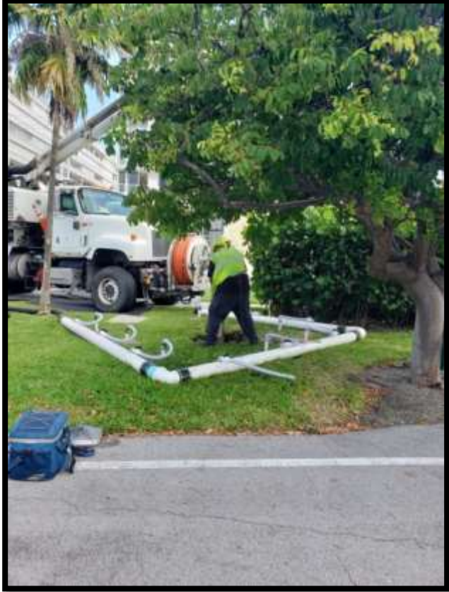
Well Point Pumping Equipment
