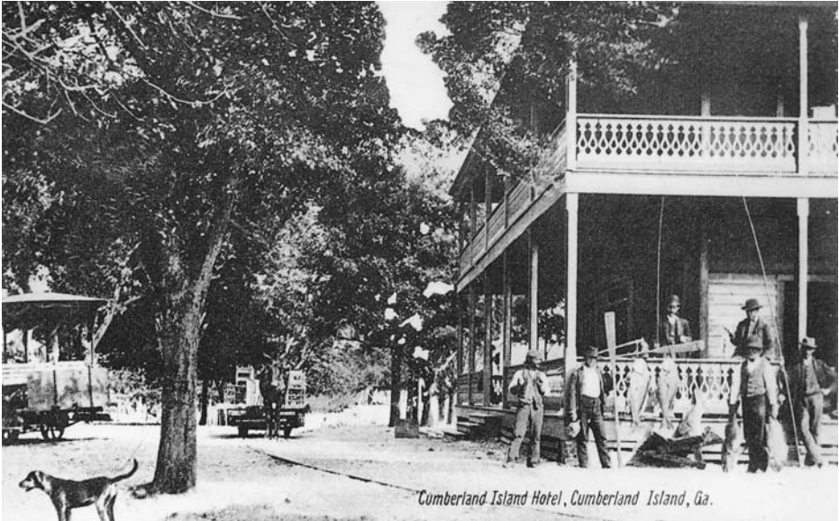
Fig. 2.11. The Cumberland Island Hotel at the north end of the island ca. 1898
