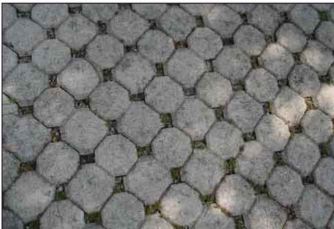
Close up of permeable paving
