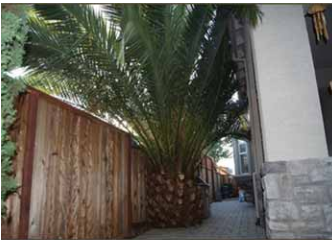
Improper placement of tree
