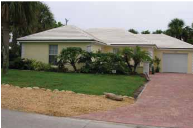
Permeable paver drive with coquina rock parking area
