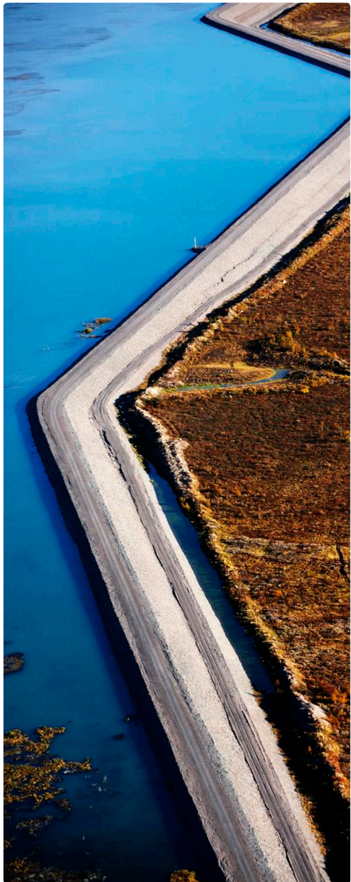
Aerial view of LKAB's dam in Kiruna.
