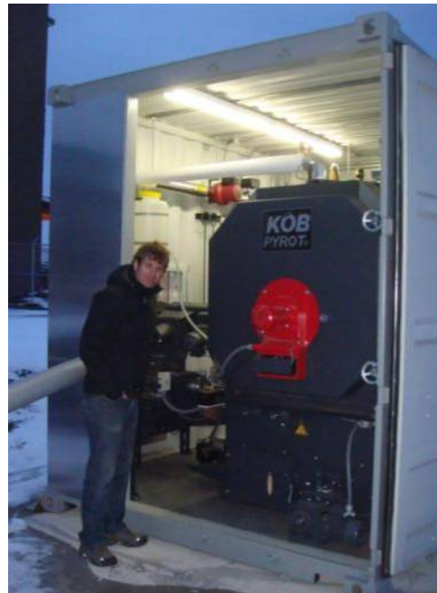
Secondary Chamber Burns Gas Heat Exchanged to Water – Flue Gas Recycled
