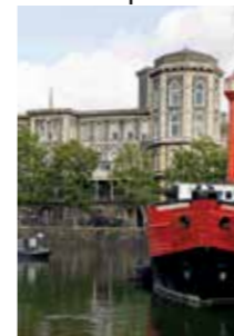
The octagonal tower without the Ogee Dome
