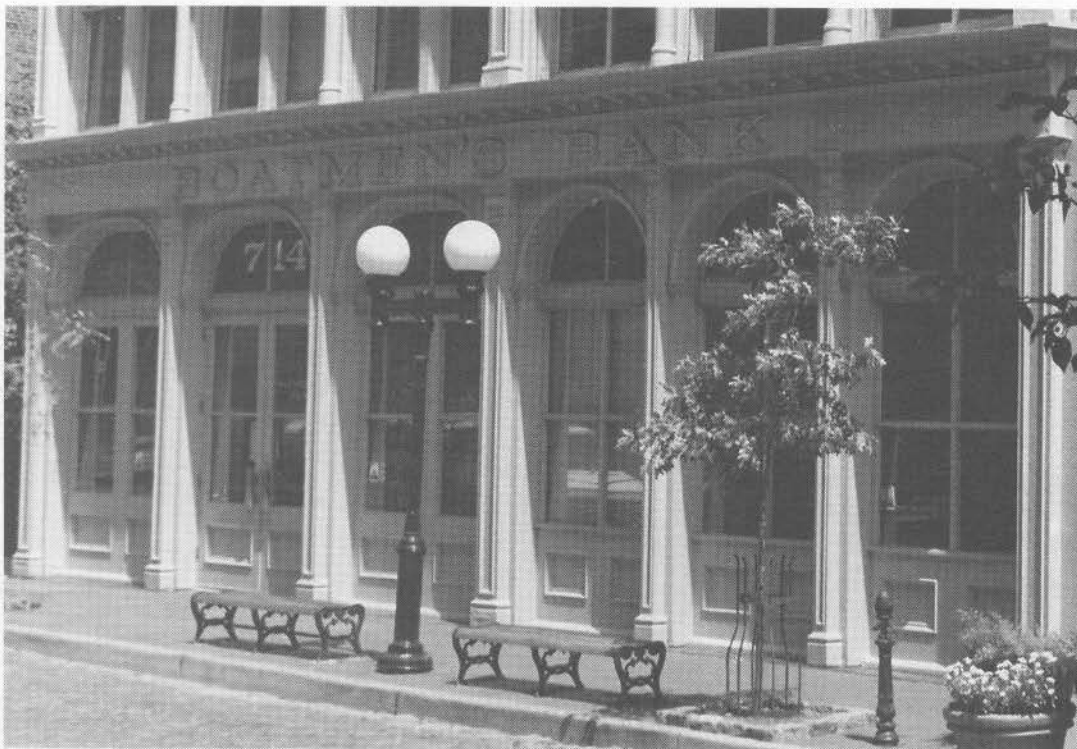
Figure 32. Ground floor of simple iron-front building at 714-16 North Second Street, just south of Morgan. Photo by Art Hebrank.
