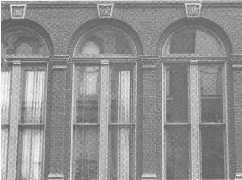
Figure 27. Cast-iron "keystones" and pilaster "capitals" complement the fancy brickwork of the second-floor facade at 720-22 North First Street. The ornate window cornices on the third floor (not in picture) are also cast iron. Photo by Art Hebrank.
