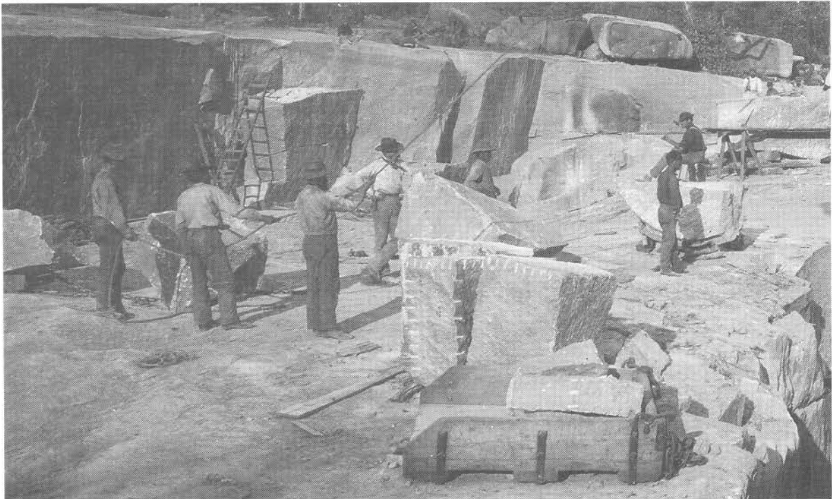
Figure 10. Granite blocks in a quarry near Graniteville, Iron County, Missouri, circa 1890. The inferior or flawed beds were broken down and hewn into "pavers." Missouri Division of Geology and Land Survey archives.
