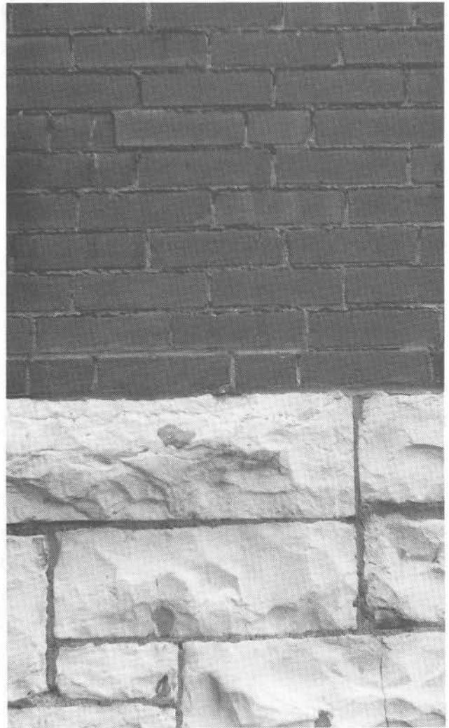
Figure 25. Common building brick on foundation of St. Louis Limestone, north side of Lucas Street just west of Clamorgan. Foundation blocks are 8 inches high. Photo by Art Hebrank.
