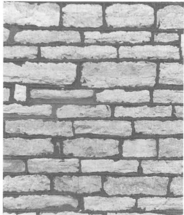
Figure 4. Rubble masonry west wall of the Old Cathedral. St. Louis Limestone rubble blocks range in height from 3 to 8 inches (same scale as fig. 3). Photo by Art Hebrank.
