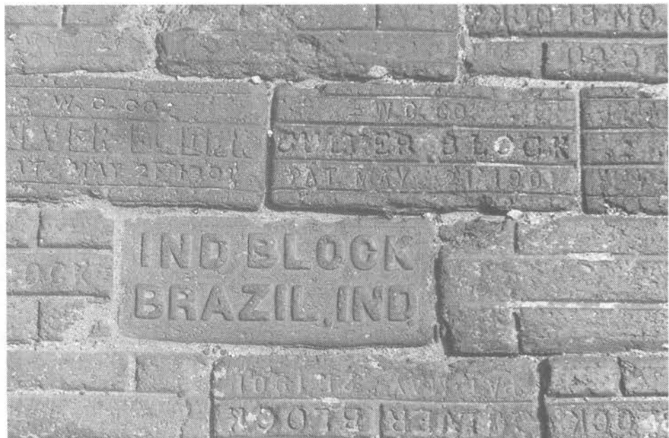
Figure 28. Detail of paving brick on Clamorgan walkway, just south of Lucas Street. Exposed faces (sides) of bricks are 9x4 inches. Photo by Art Hebrank.
