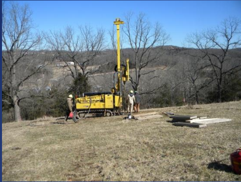
Drilling the feature in 2010
