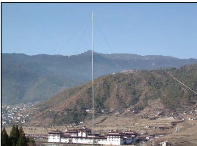
A51B 80m vertical: This is at A51AA’s QTH, where I was EVERY evening for gray line. This is a Gladiator top-loaded vertical on a mountainside, overlooking the Thimphu Dzong (the national capital building).
