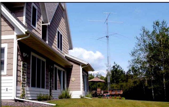
Don’s back yard and 72 ft. crank-up with Titanex LPDA and Force-12 30/40 meter combo on a Tic Ring rotor.
