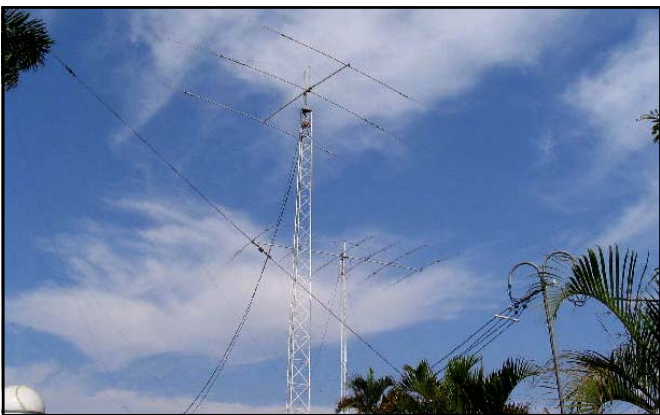
Towers with WARC band antenna in foreground and KLM tri-bander in the background.
