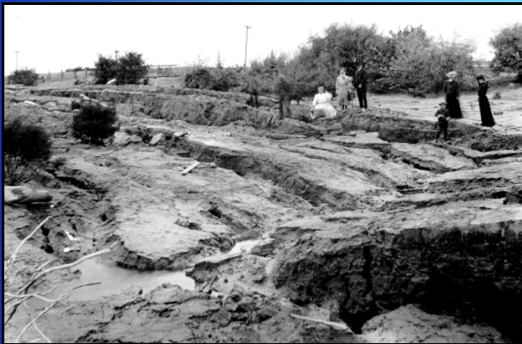
Bank failure on the Eel River near Port Kenyon due to liquefaction.
