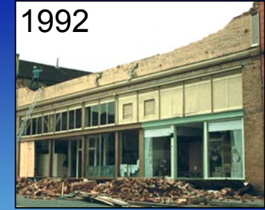
393 Main St. in Ferndale suffered similar damage in the 1992 and 1906 earthquakes. However more of the parapet wall fell and all of the windows were broken in 1906.
