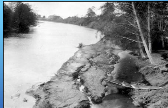
Liquefaction on the banks of the Salt River.
