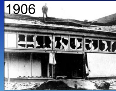
393 Main St. in Ferndale suffered similar damage in the 1992 and 1906 earthquakes. However more of the parapet wall fell and all of the windows were broken in 1906.
