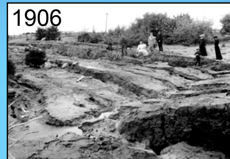
Liquefaction was observed along the Mattole River (above left) and locally in the Eel River Valley in 1992. In 1906 it was much more dramatic and widespread.
