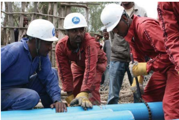
Practical exercise in Drilling Technology Course. Constructed wells are used as production wells.
