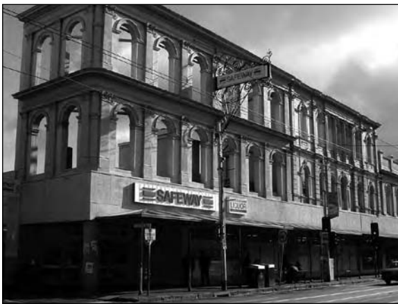
Facadism resulting from inadequate fabric retention
