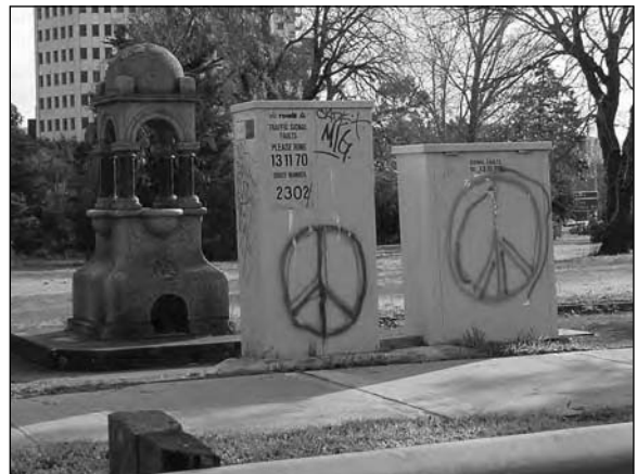
Inappropriate placement of modern services close to Contributory Elements of a Heritage Place
