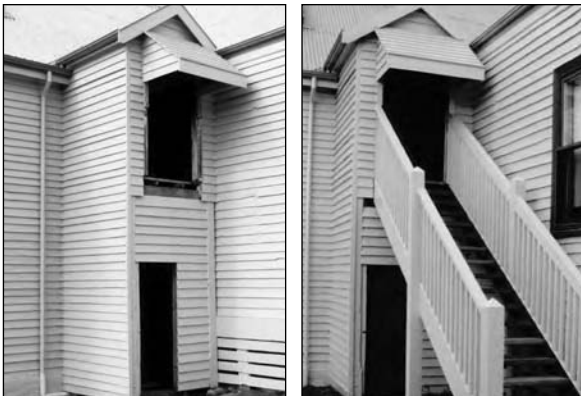
Reconstruction of the rear stairwell of the Toongabbie Mechanics Institute – before (left) and after reinstatement of missing parts (right)
