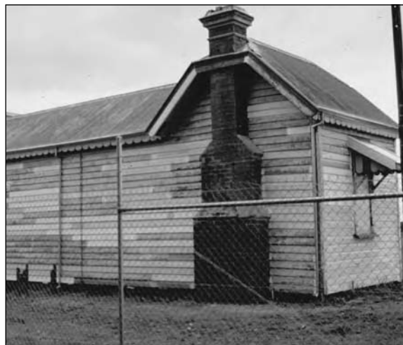
Most Heritage Places are able to be repaired: Pirron Yallock Railway Station before (top) and after repair (below)
