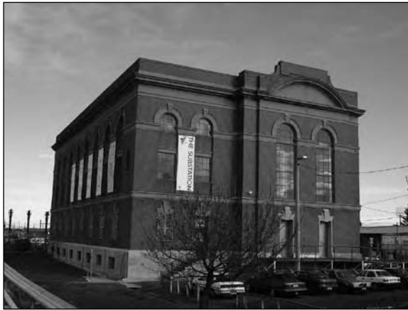
Adaptive reuse of an industrial Heritage Place: the former Newport Railway Electricity Substation undergoing conversion to a community arts centre
