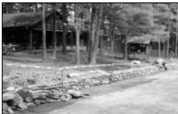
Wall project nears completion for camp
