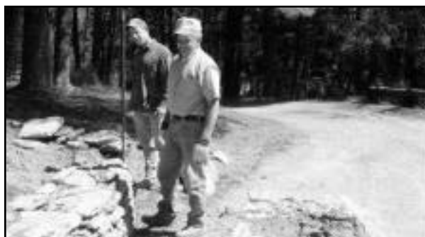
Work progresses on new wall steps
