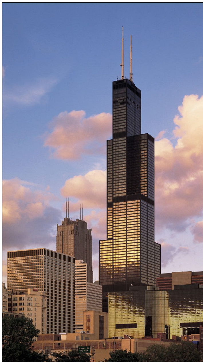
The Willis Tower might look sleek and black on the outside, but it's quite "green" on the inside.
