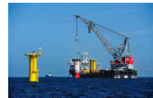
Building of the offshore wind farm Riffgat.
