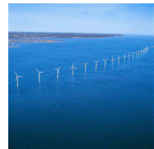
Middelgrunden offshore wind farm. © Siemens press image
