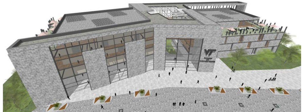
Figure 2: Case Study #2 Office Building
