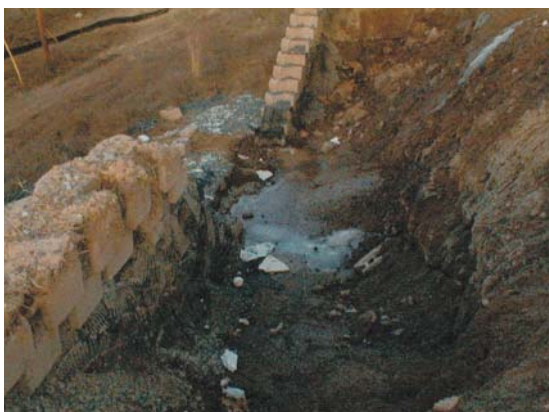
Fig. 8 Groundwater exiting from retained soil zone in cut-situation (authors)
