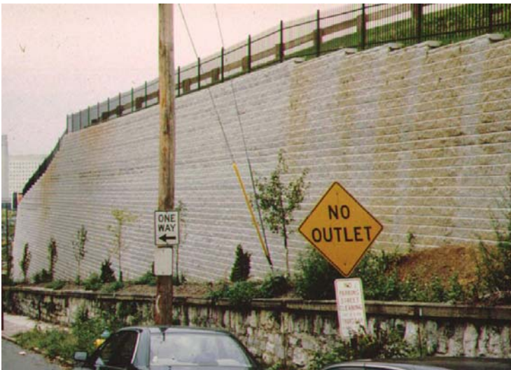
(b) Masonry block, also called segmental retaining walls, faced wall
