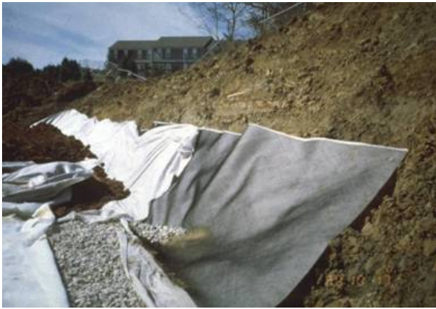
(c) Use of continuous and intermittent geocomposite back drains when using fine grained soils in the reinforced soil zone (compl., TenCate Geosynthetics, Inc.)
