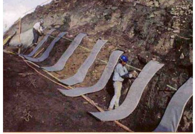
(c) Use of continuous and intermittent geocomposite back drains when using fine grained soils in the reinforced soil zone (compl., TenCate Geosynthetics, Inc.)
