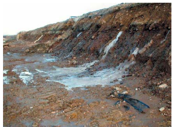
Fig. 8 Groundwater exiting from retained soil zone in cut-situation (authors)
