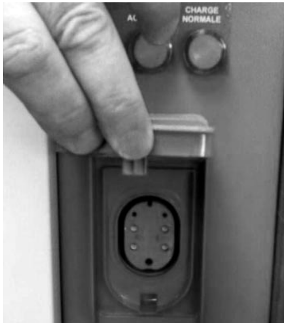
Figure 16.4 Type 3 plug on one of the first EVplug alliance charging station, deployed in France.
