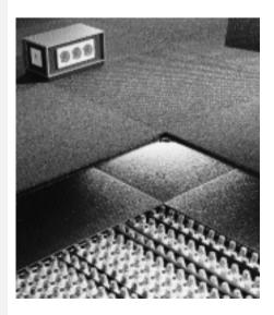
Such a structure made of polyester or glass yarns is coated and moulded into a light-weight three-dimensional and extremely tough "honeycomb" construction.
