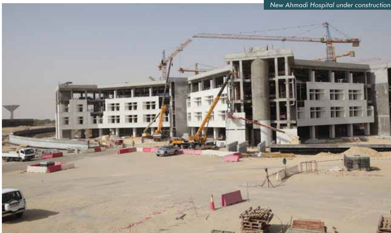
New Ahmadi Hospital under construction.
