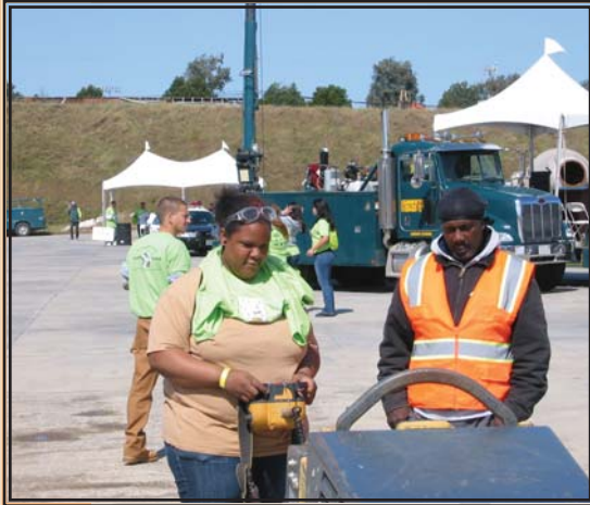
Willie Robertson (R) of the Laborers' Training Center demonstrates the operation of a wireless remote roller.
