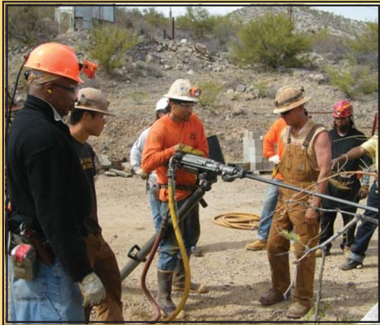
Terrone Hart practicing drilling holes outside for blasting or ground support.
