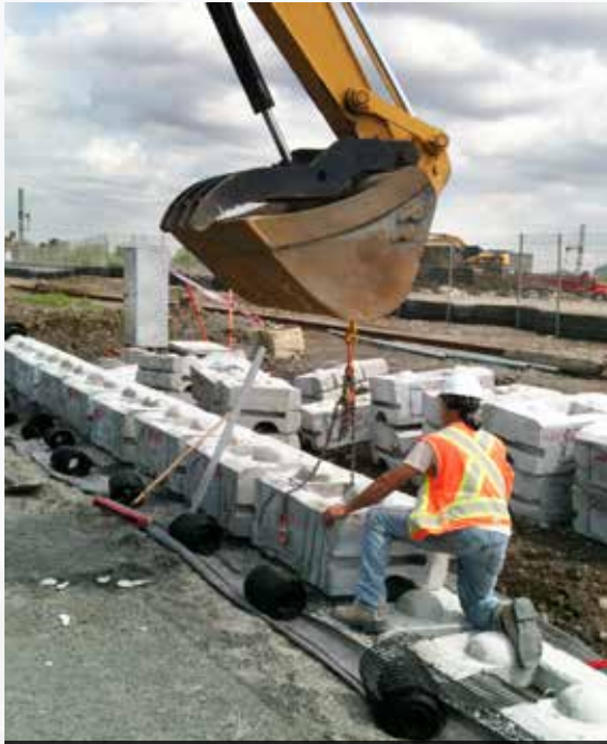
Each Redi-Rock block installs like a massive Lego block using a piece of heavy machinery and a small crew. This efficient installation process results in saved time and money.
