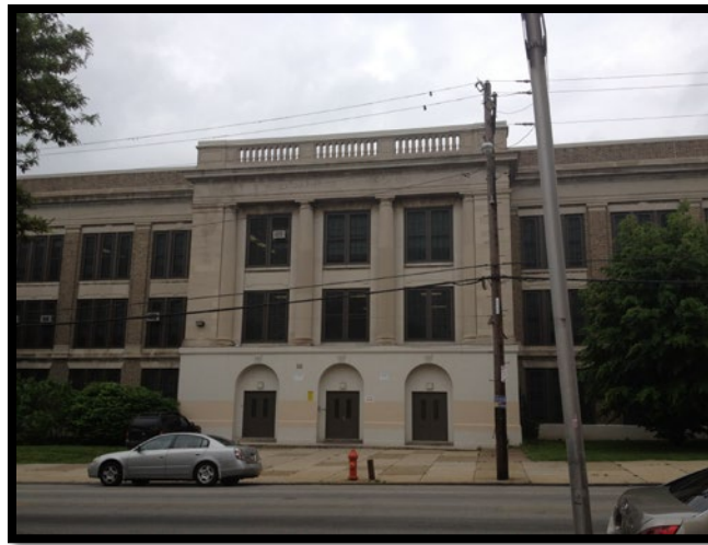
Figure 7 Mayer Sulzberger Middle School
