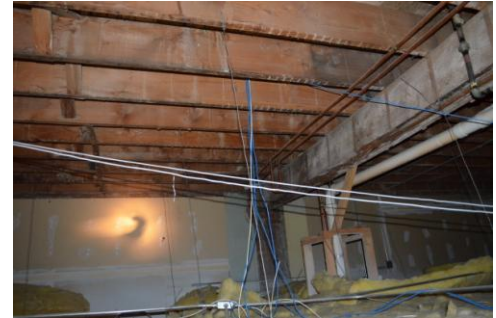
Floor Joist & Dropped Beam
