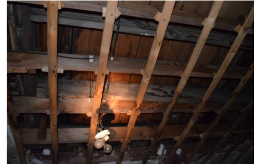
Exposed Roof Rafters and Ceiling Joists
