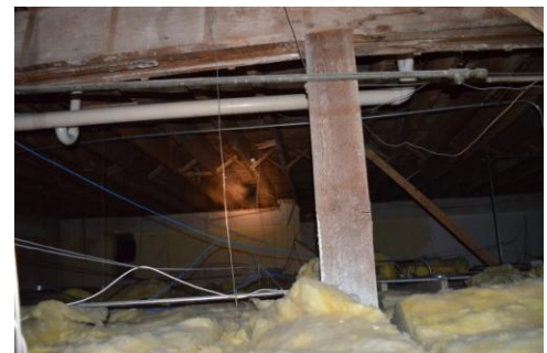
Beam Bearing at Timber Column
