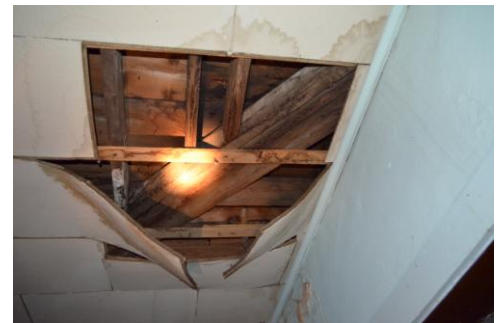
Diagonal Beam at Corner of "U-Shape" Area
