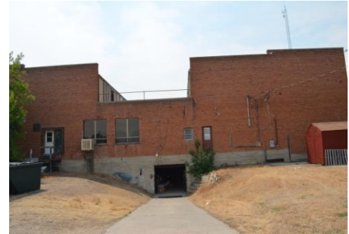
Visible Foundation Wall at North Elevation
