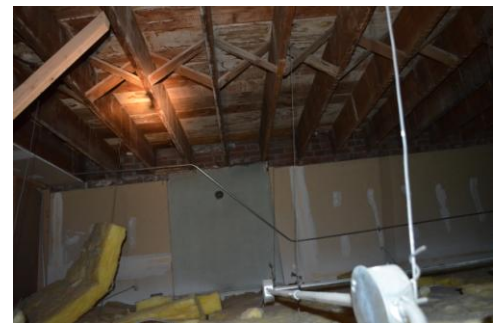
Joist Blocking
