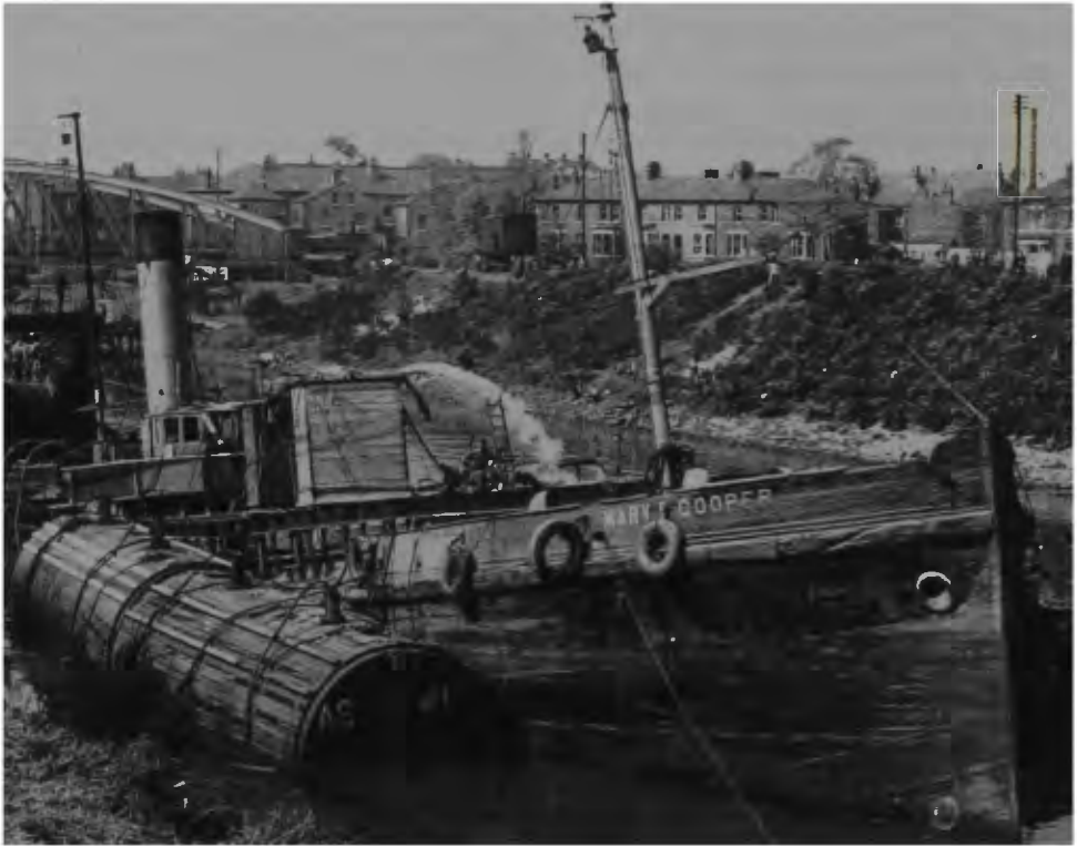
The Mary P. Cooper was successfully raised on 16 th April, 1961
