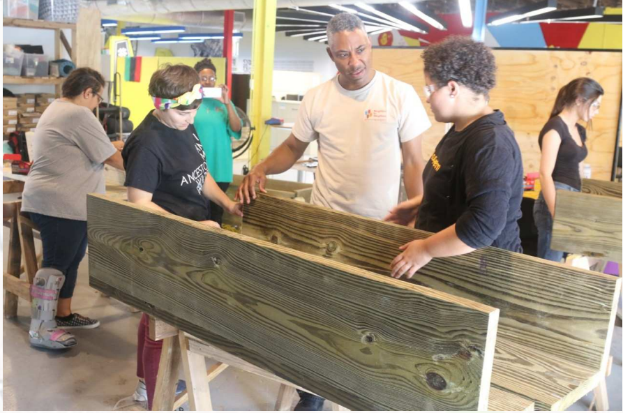
September 11 Day of Service Build Day at Six Points Innovation Center.
