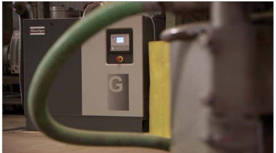
An Atlas Copco GHS VSD+ vacuum pump. Industrial vacuum pumps are used in a wide variety of applications.
