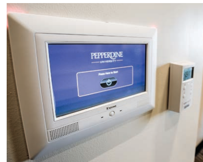
Touchpanels were selected to replace the originally specified button-touch control panels. The choice better reflects a millennial predilection for touchscreens.
