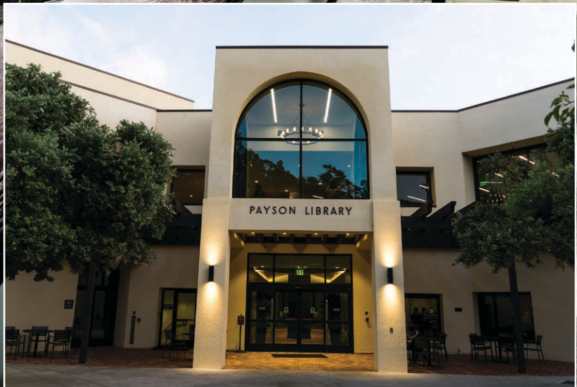
The Payson Library reopened in September 2017 after an $18.8 million renovation of the 71,000-square-foot building was completed. The renovation included significant AV systems integration.
