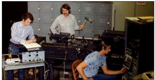
Figure 14. Impact test of lathe, student project group: Chris Powell, Randy Allemang and Tom Graef, left to right (1972).
