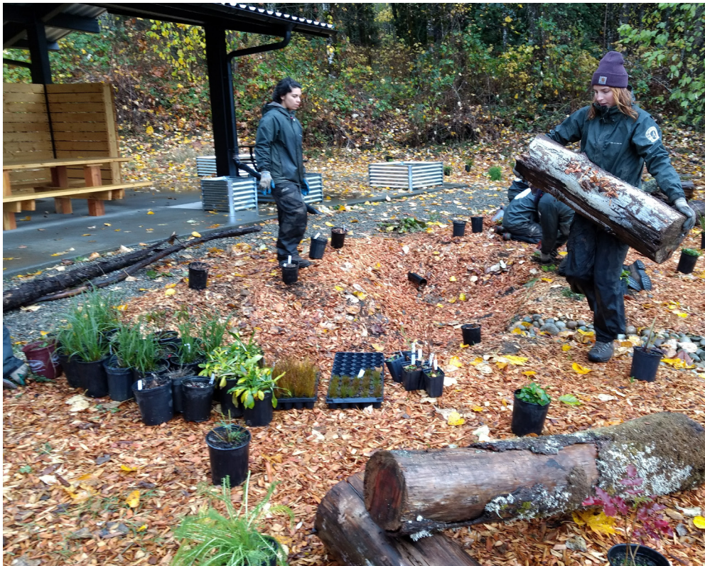
Figure 21. Placing woody debris and planting flowering herbaceous plants at a rain garden installation in Woodinville, WA.
