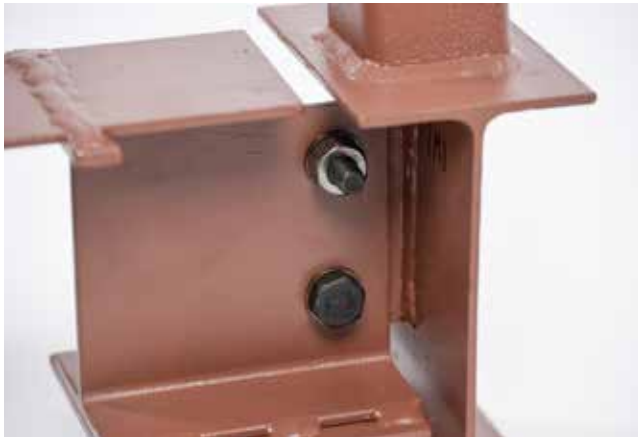
▲ SSS: Bolt head orientation not defined.
