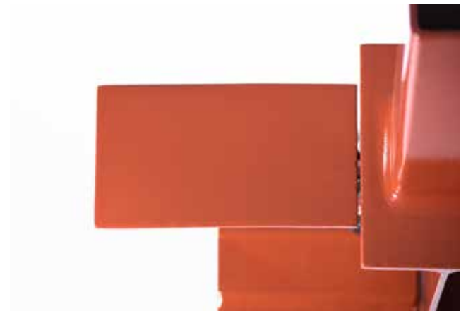
▲ AESS 4: Surfaces filed and sanded.
