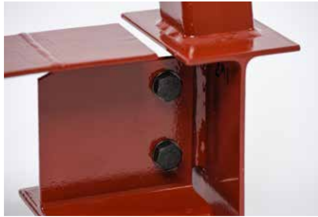
▲ AESS 1: Bolt head orientation defined, backing bar removed.
