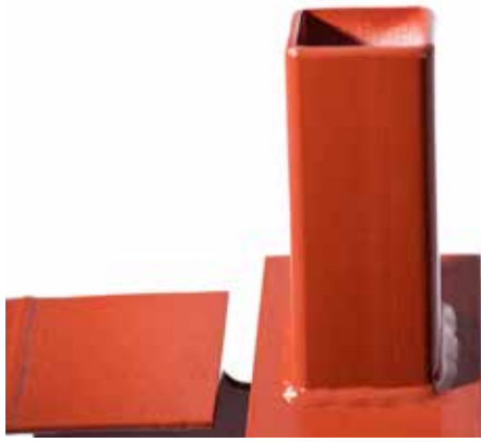
▲ AESS 2: HSS weld seam orientation not defined.
