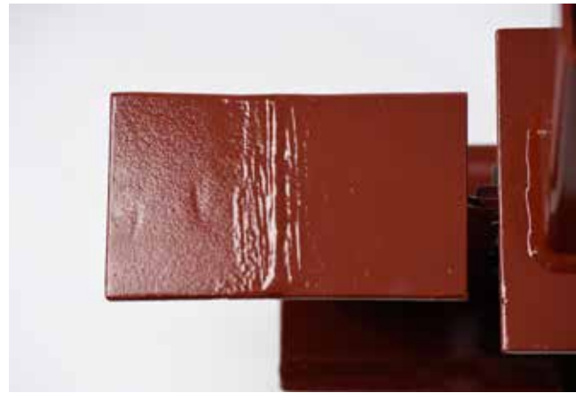
▲ AESS 1: Welds uniform and smooth and backing bars removed.
