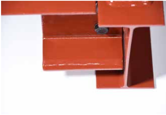
▲ AESS 3: A contoured weld.
