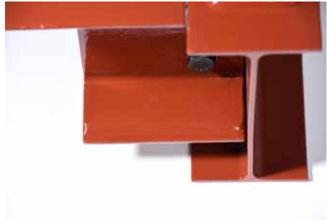
▲ AESS 4: In addition to a contoured and blended appearance, weld transitions also are contoured and blended.
