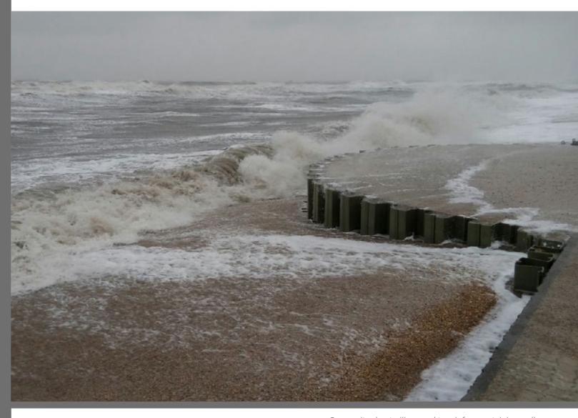
Composite sheet piling used to reinforce retaining walls.
