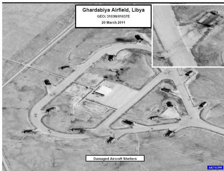
Figure 11: Aircraft Shelters at Ghardabiya Airfield, Libya, after a B-2 Strike, March 20, 2011 71
