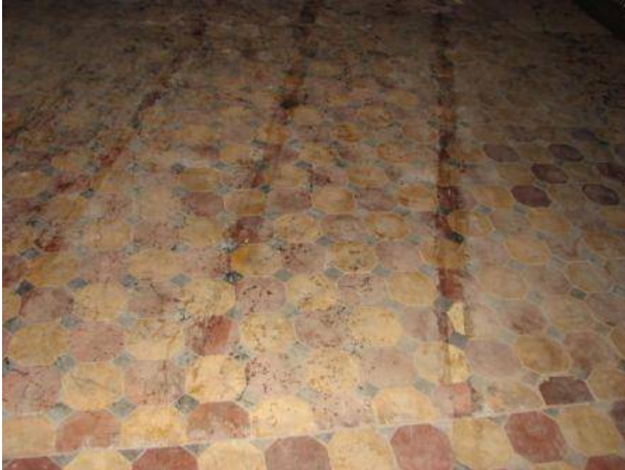
Basement floor tiles as they looked in Jun3 2008
