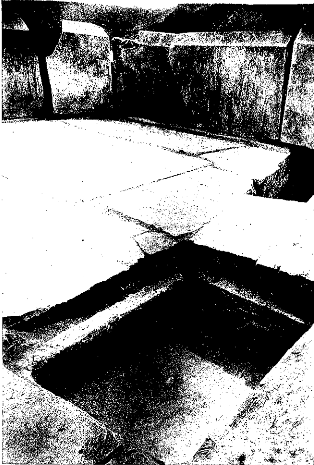
LEAD TANK OF DRAIN.
